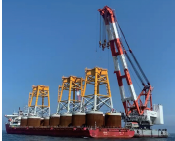
Figure 1 Jacket foundation of an offshore wind turbine
