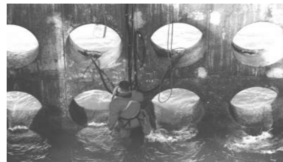
Fig. 2 Perforated wall breakwater of Dieppe, France, in Bêlorgey et al. (2003)
