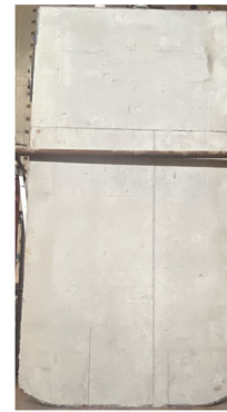
Fig. 12 Overall failure mode of specimen RW-1
