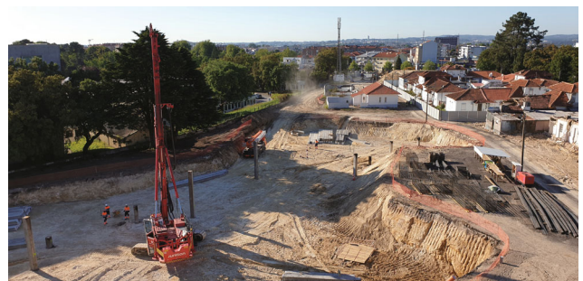
Fig. 4 General view of the experimental test site
