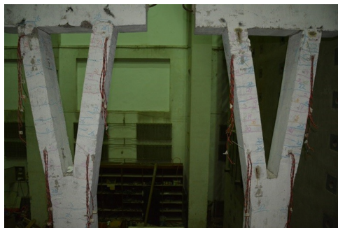
Fig. 33 Damage of the top of columns
