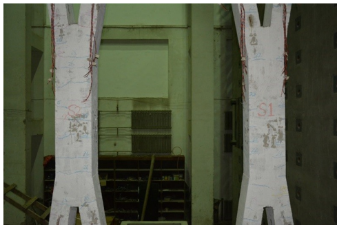
Fig. 34 Damage of the middle of columns
