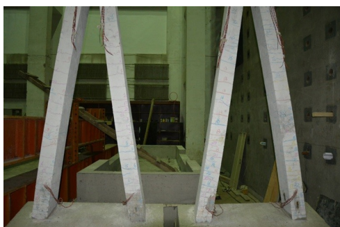
Fig. 35 Damage of the bottom of columns
