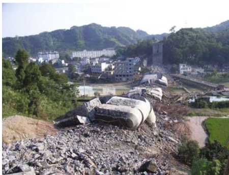
Fig. 13 Collapsed bridge over Dixituo River
