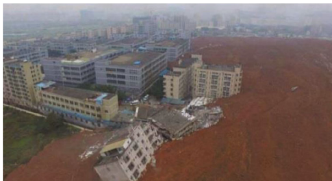
Fig. 7 Buildings in Shenzhen buried by landslide in December 2015 (Source: Baidu Baike)
