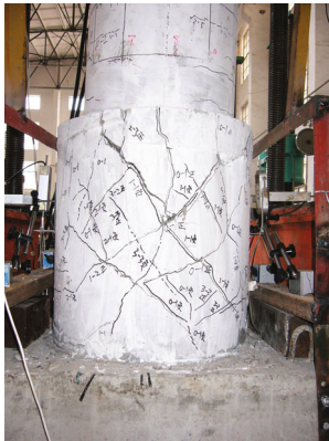
(a) Vertical and diagonal cracks of the concrete jacket
