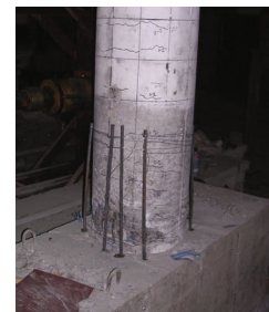
(b) Specimen A10 after installation of additional longitudinal bars
