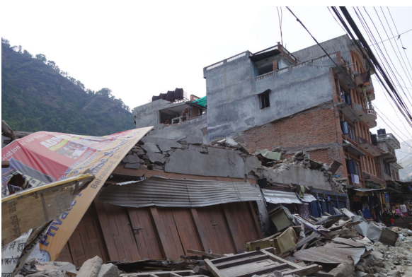
Fig. 4 Complete collapse of a rubble structure in Intensity IX area
