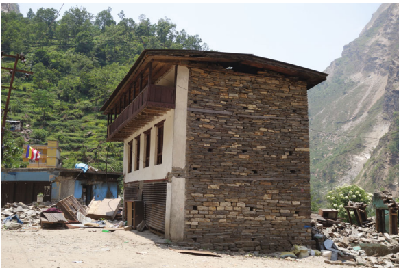
Fig. 2 Typical rubble structure
