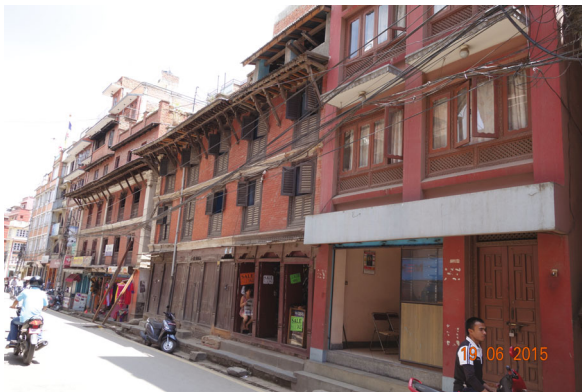
Fig. 10 Traditional brick-wood structure in the city of Katmandu
