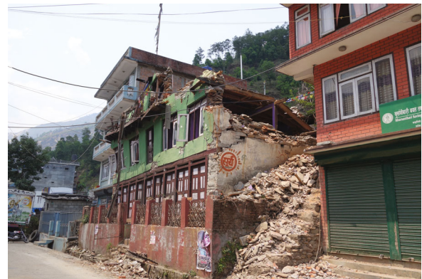
Fig. 3 Partial collapse of a rubble structure in Intensity VIII area
