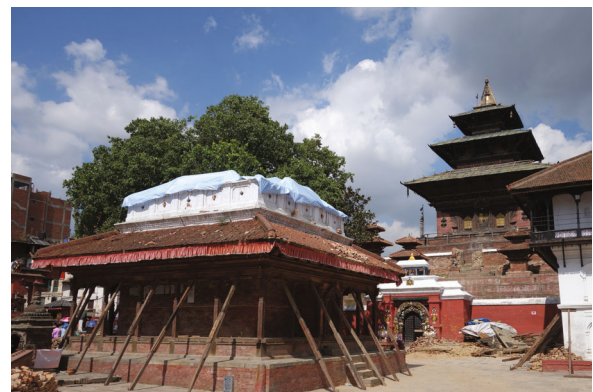
Fig. 15 Collapse of the temple in Durbar Square, Katmandu
