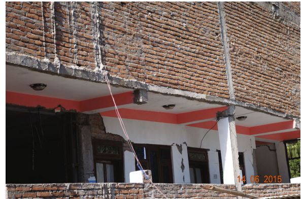
Fig. 7 Frame column cast into the bottom of the frame beam
