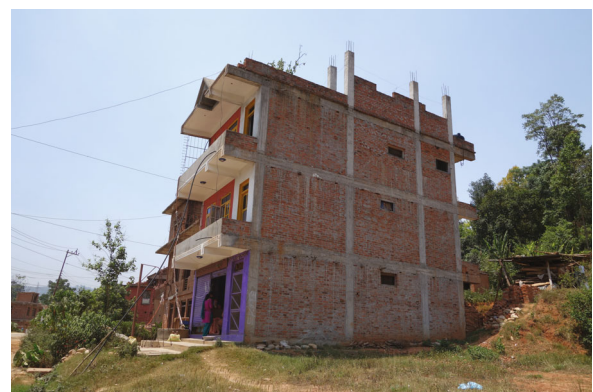
Fig. 5 Typical RC frame structure
