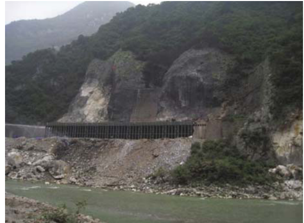
Fig. 8 Landslide damaged railway, sealed tunnel and caused fire of oil train
