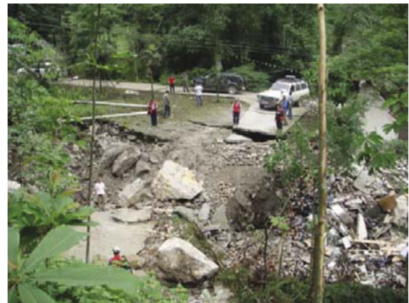
Fig. 3 A big vertical dislocation of 4.7m in Hongkou Town, showing strong thrust movement of the Longmenshan fault
