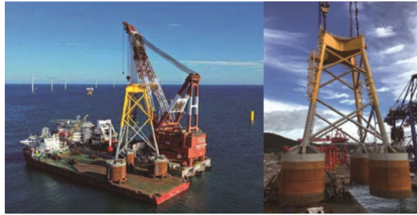
Fig.1 Multi-bucket jacket foundations for OWTs in China.
