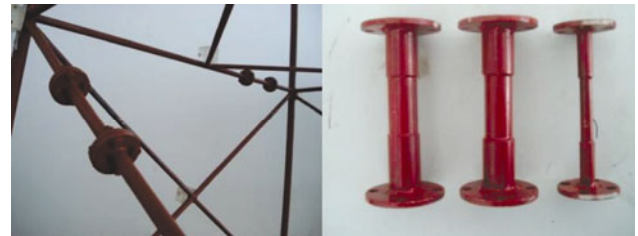
Fig.7 Replacements for damage simulation.
