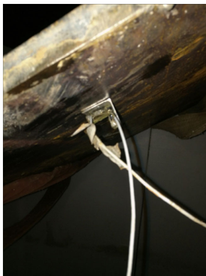
Figure 5 Acceleration sensors in steel plate
