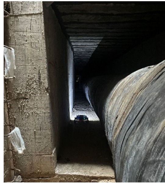
Fig. 1 Underground Tunnel with Pipelines
