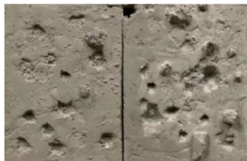
(a) Concrete Walls
