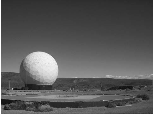
Figure 1. The single geodesic radome remaining at the former NSA early warning facility at Nurrungar, near Woomera. Note the footings of other dismantled radomes at the same site
