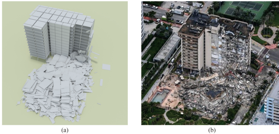
Fig. 15 Comparison between simulated and actual collapse wreckage (photo via Agence France-Presse). (a) Simulated collapse wreckage; (b) actual collapse wreckage.
