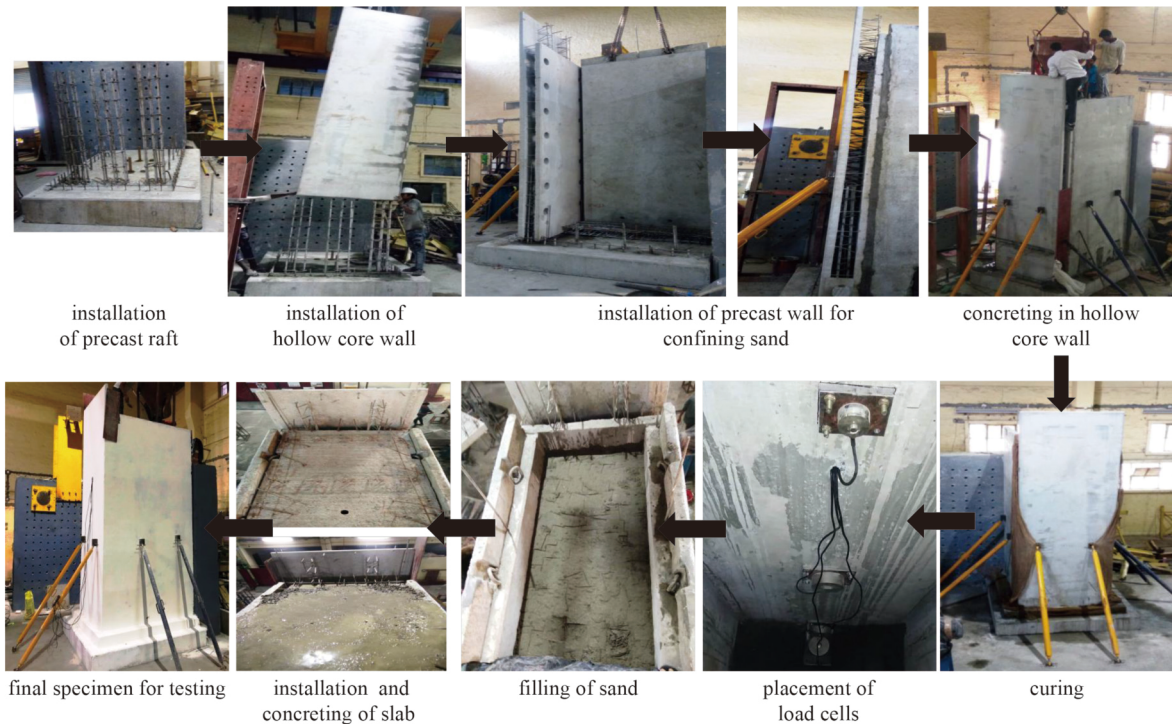
Fig. 2 Installation of PDLs in laboratory.
