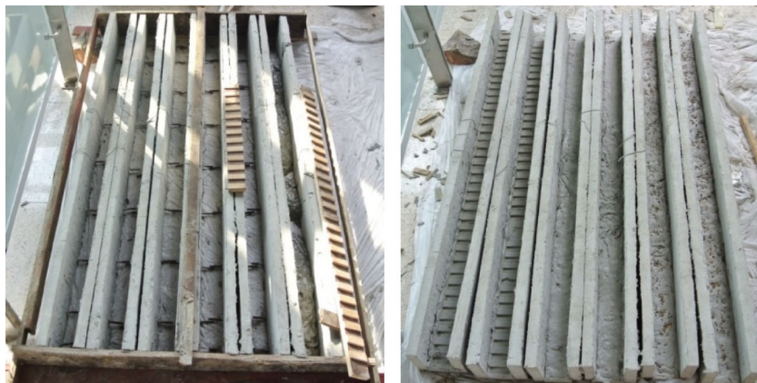
Fig. 3 Fabrication of the ECC permanent formwork.
