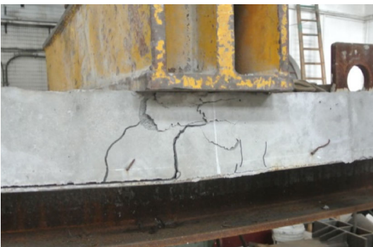
Fig. 5 Failure mode of specimen S-2
