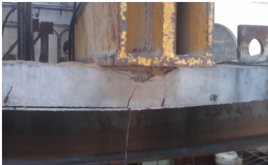
Fig. 4 Failure mode of specimen S-1
