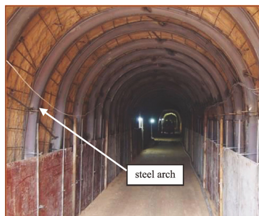
Fig. 1 Steel arch used in tunnel engineering
