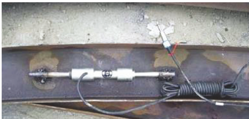
Fig. 7 Strain gauges installed in field
