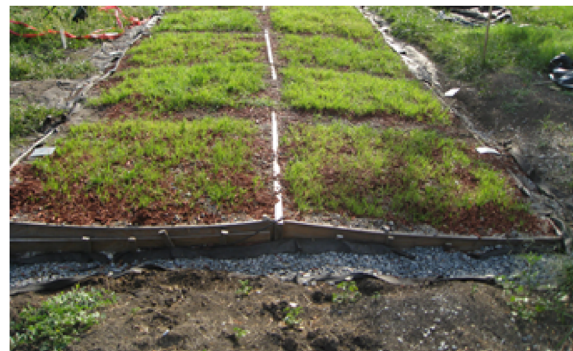
Fig. 11 Geocell-stabilized unpaved shoulders [42]
