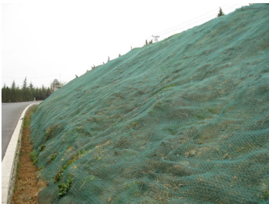
Fig. 6 Geosynthetic erosion mat-protected slope (photo taken by J. Han)
