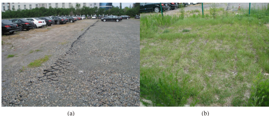
Fig. 12 Geocell-stabilized gravel versus vegetated parking lots (photo taken by J. Han). (a) Gravel parking lot; (b) vegetated parking lot
