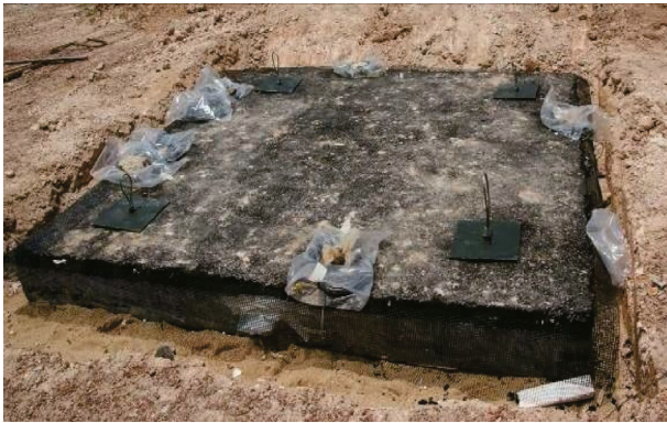
Fig. 17 Completed SHS multi-layer composite slab with anchoring at site
