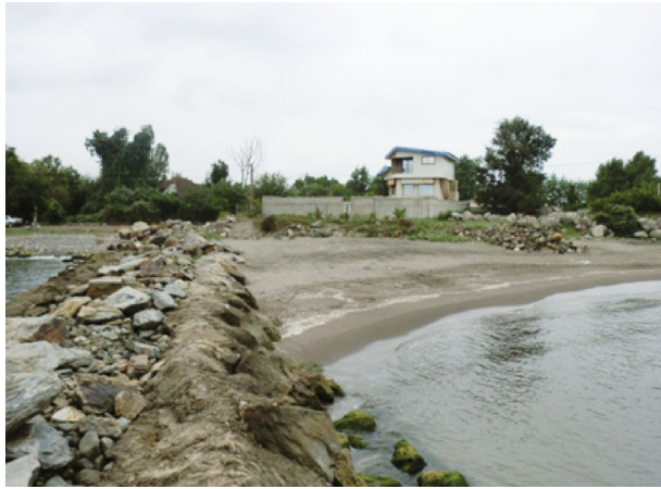
Fig. 17 Beach deformation in the vicinity of groyne at Dahane Sar Sefidrood
