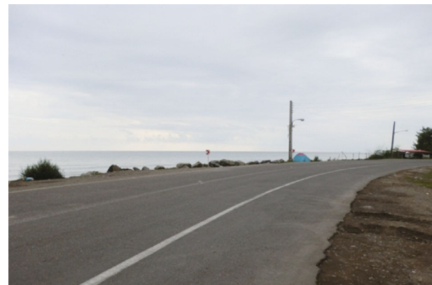
Fig. 3 Coastal road exposed to waves
