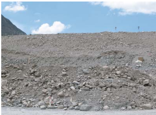
Fig. 2 Rockfill dam – Caracoles Dam
