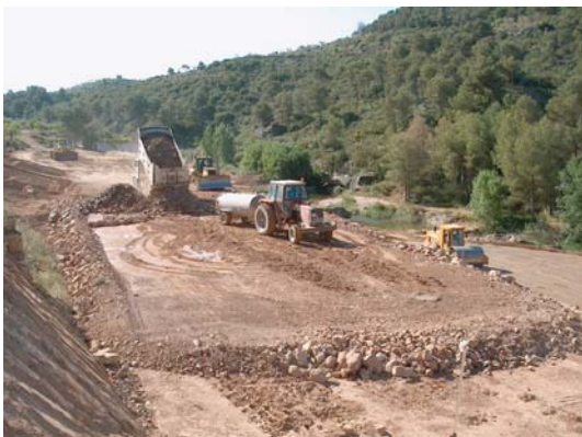
Fig. 3 Construction of a trial embankment for Albagés Dam
