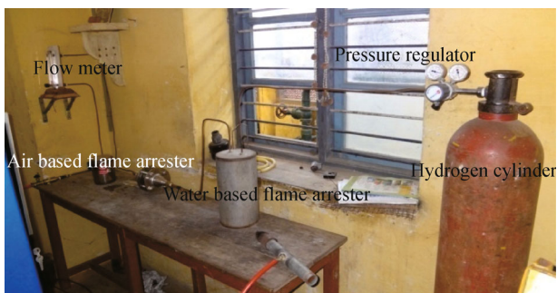
Fig. 5 Hydrogen flow line
