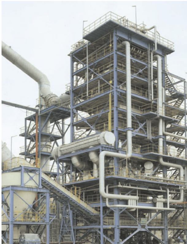
Fig. 14 Waste heat recovery boiler [109]
