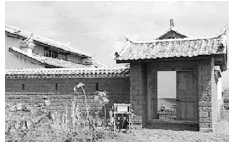
Fig. 12 The first new rammed earth house built as a demonstration
