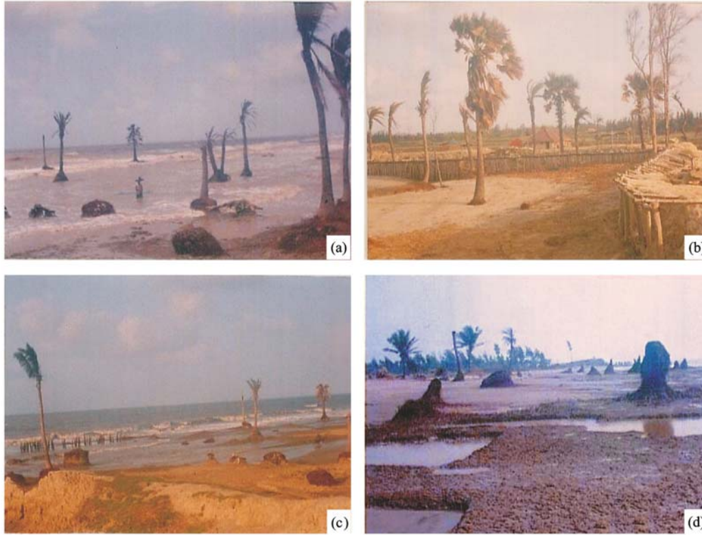
Fig. 3 Field photographs showing beach erosion at Sagar Island: 3(a) Beach erosion; 3(b) Mud embankment with bamboo poles to prevent beach erosion; 3(c) Beach erosion showing remnants of tree roots; 3(d) Remnant of mud bank exposed on the beach
