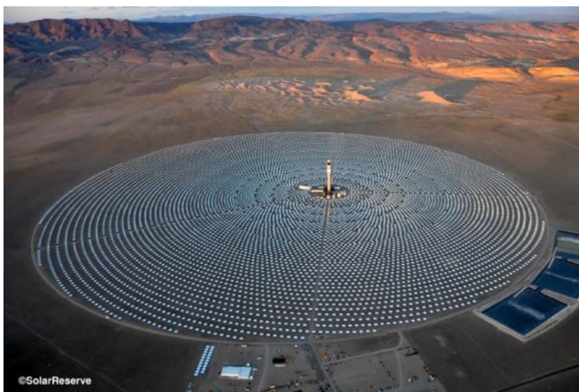
Fig. 2 110-MWe Crescent Dunes tower CSP plant in Tonopah, Nevada, USA, with 10 h of thermal storage in ~32000 tons solar salt (source: SolarReserve)
