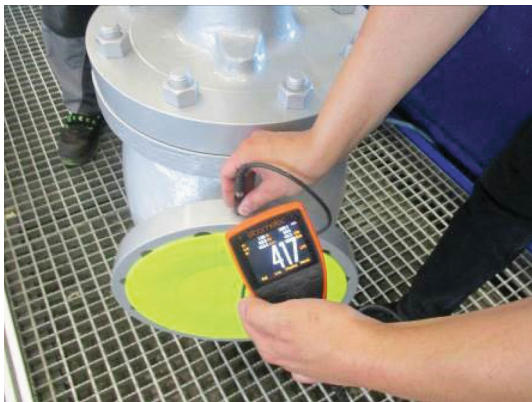
Fig. 4 PMI test on a 22Cr duplex gate valve in EG project
