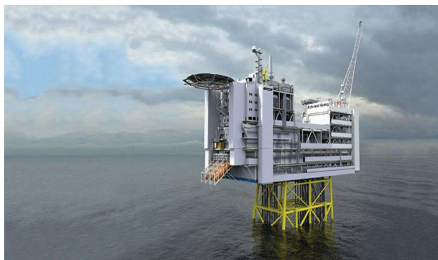
Fig. 3 Edvard Grieg Field after Jacket Installation
