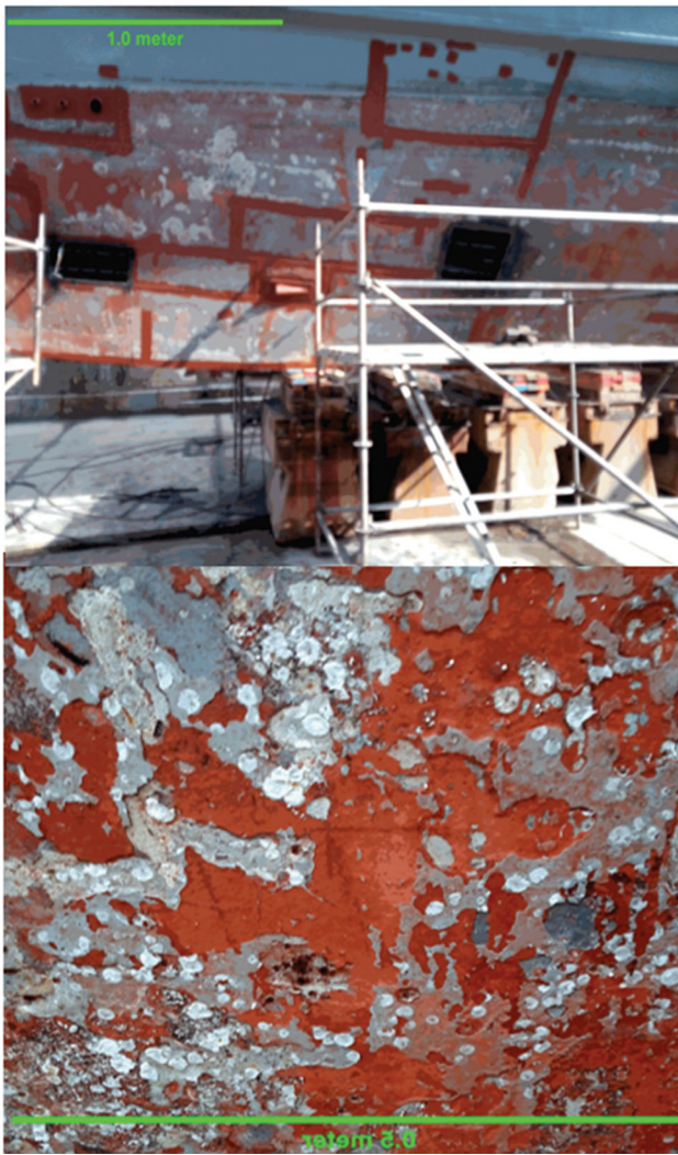
Fig. 2 (a) Removal of samples from damaged ship hull (b) pitting corrosion on the surface of the steel
