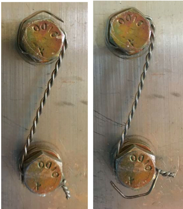
Fig. 3 Safety wired bolt assemblies after safety lock wire failure
