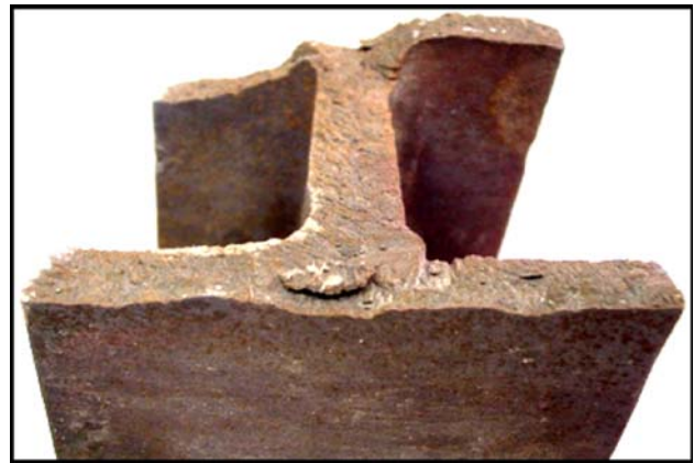
Fig. 1 Fracture surface of one of the furnace tube support samples-HK-40
