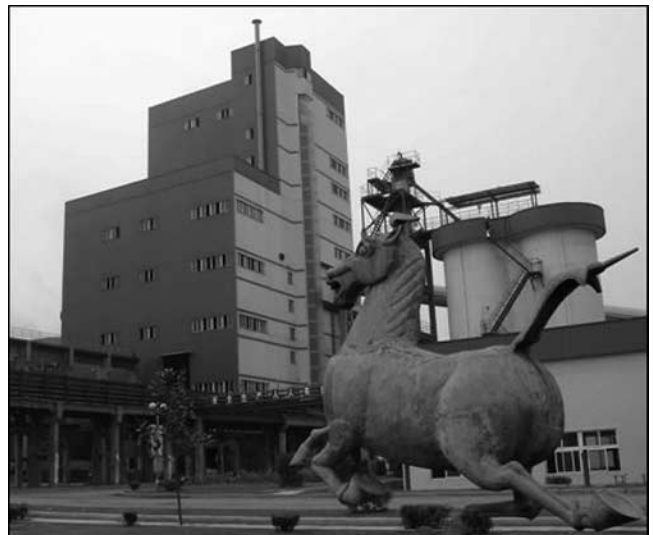
Fig. 17—Ausmelt copper smelter at Anhui Tongdu Copper (Tongling City, China).
