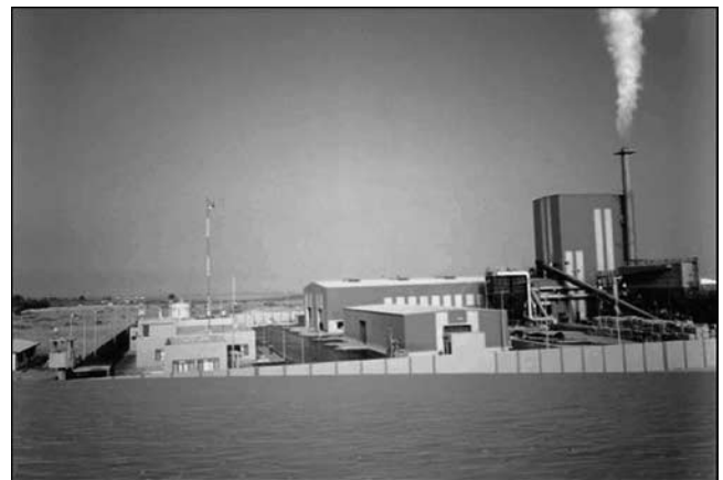
Fig. 19—View of the Funsur tin smelter and the control room during operations.
