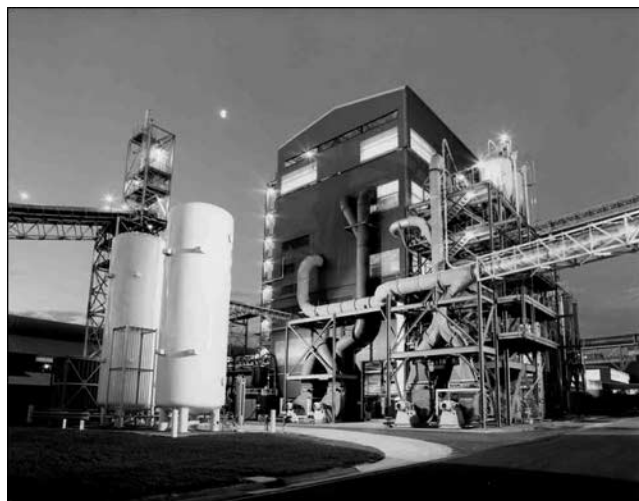
Fig. 21—SPL Recycle Plant at Portland Aluminum/Alcoa (Australia).
