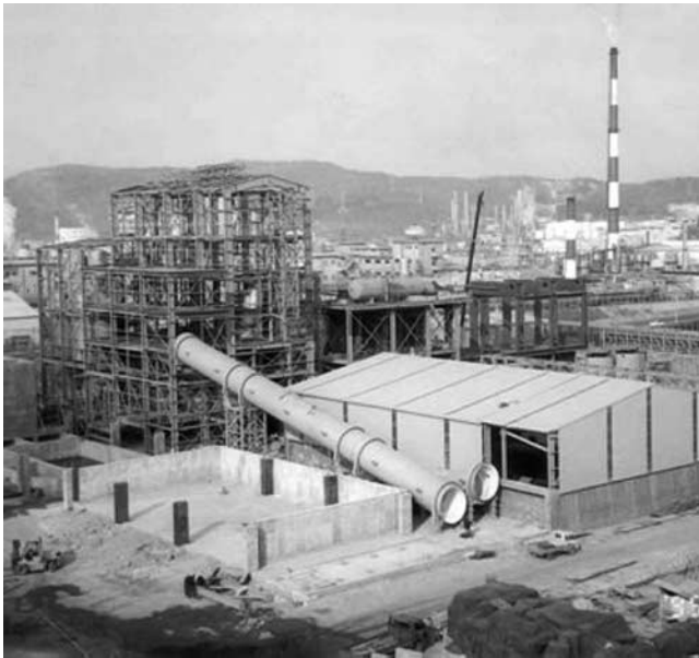
Fig. 14—Korea Zinc Co. Residue Fuming Plant during construction.
