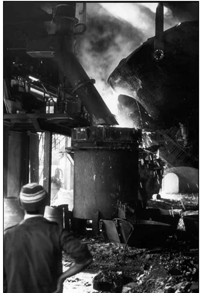
Fig. 9—Filling the ER&S 1-ton plant with liquid-copper converter slag.
