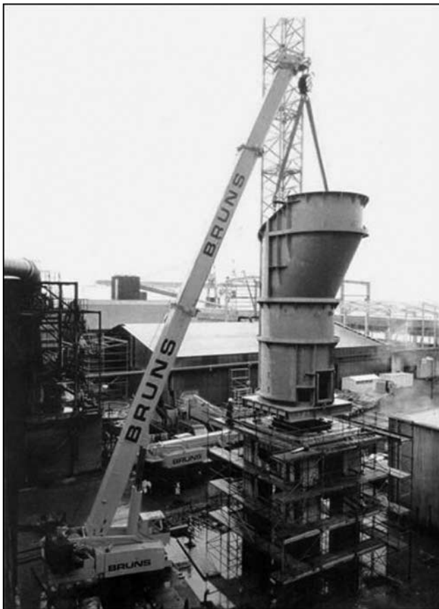
Fig. 18—Lead smelter, Metaleurop (Nordenham, Germany) during construction and on the operating floor during smelting of lead concentrates and battery paste.
