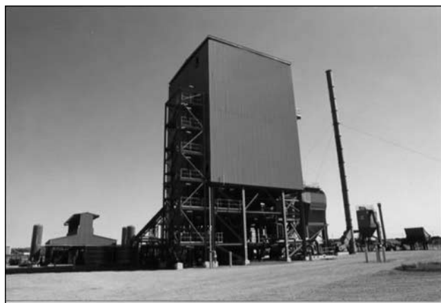
Fig. 22—Iron ore to pig iron demonstration plant (Whyalla, South Australia).
