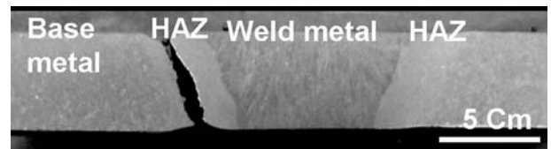
Fig. 6—Location of creep failure in the 9Cr-1MoVNb steel weld joint.
