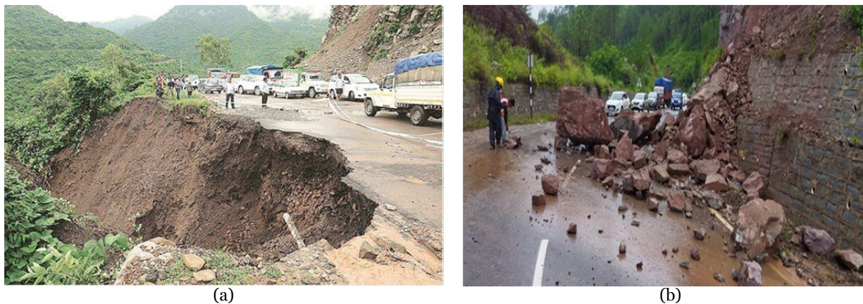
Fig. 10 Landslide damage on NH 5. (a) A portion of Parwanoo-Shimla road caved near Chakki Mod (Source: https://indianexpress.com/article/india/landslides-disrupt-rail-and-road-traffic-between-chandigarh-and-shimla-5305537/ ); (b) Big boulders often fall on the four-laned Parwanoo-Dharampur section (https://www.tribuneindia.com/news/himachal/single-lane-traffic-to-avert-mishaps-on-parwanoo-nh-301197).
