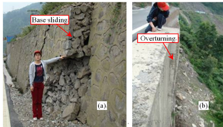
Figure 11 Deformation modes of retaining walls on soil foundation (a) and rock foundation (b).
