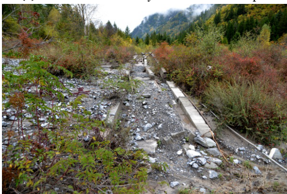
(c) Damaged tourist facilities by debris flow
