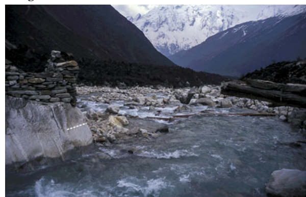
Figure 10 Photo 6 on April 20, 2008, at measurement point 9 at 3520 m a.s.l., facing southeast: The bridge was destroyed by an avalanche surge on April 20, 2008. The weathering effects and erosional processes on the boulder (---) are indicative of past floods.
