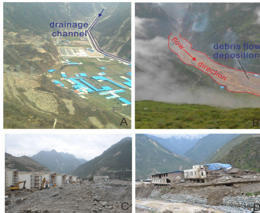
Figure 5 (A) a few buildings of local residents and factories located in the downstream gully before the 11 July debris flow event; (B) almost all the buildings were destroyed after the 11 July debris flow event; (C), (D) debris deposition on the alluvial fan and buildings destroyed by the debris flow.
