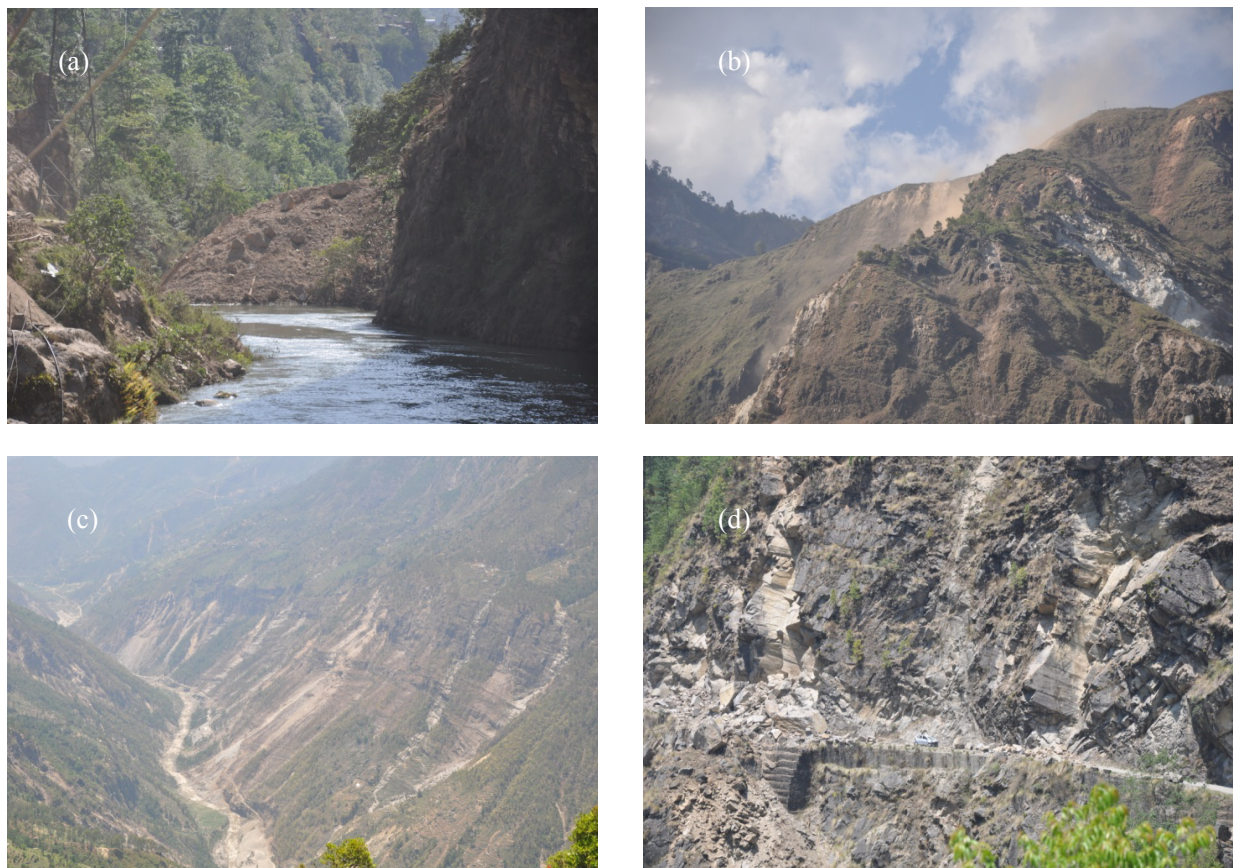
Figure 4 Photographs of some landslides taken immediately after the Gorkha earthquake. (a) Partial damming of the Bhote Koshi River due to a coseismic landslide (debris slide); (b) Smoke of dust flowing into the air due to a sliding mass; (c) Several shallow landslides observed along Trishuli River on the way to Rasuwagadi from Nuwakot after the earthquake; (d) Rock fall along the Kathmandu-Rasuwagadi road section completely blocking the traffic.
