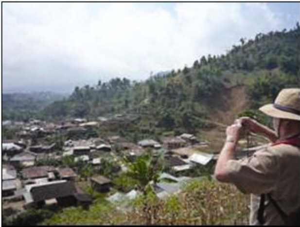
Figure 4 Un-appropriate landuse management, where many houses of situated immediately at the lower part of susceptible slope.
