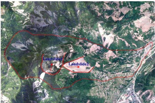
Figure 3 Landslides in debris-flow source area
