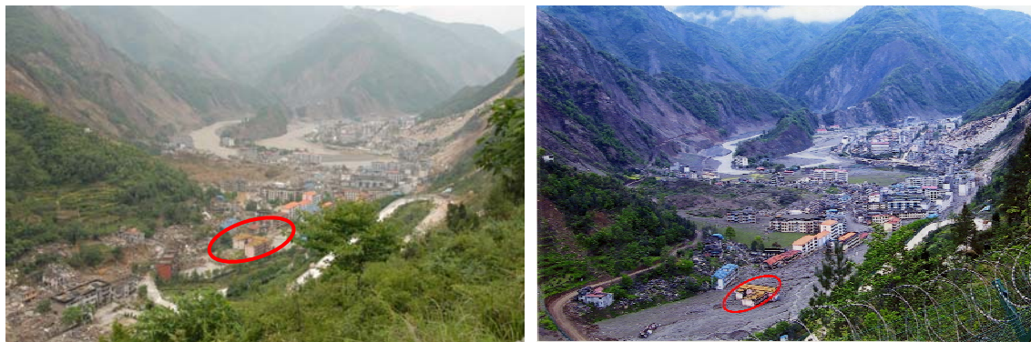
Beichuan township after the quake before debris flow occurrence
