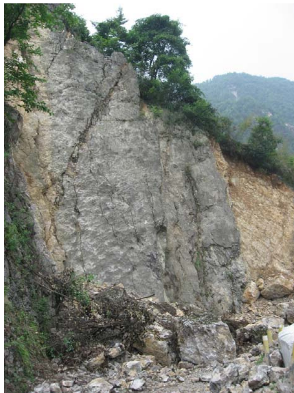
Figure 4 A steep rock slope with fully developed cracks
