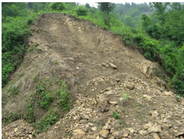
Figure 2 Shallow failure of soil slope
