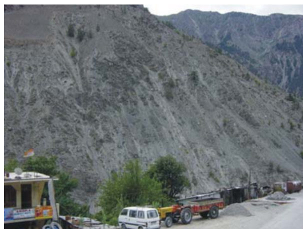
Figure 12 Unstable hill slope showing the initiation of landslide near Spilo in the Morang-Pooh section.
