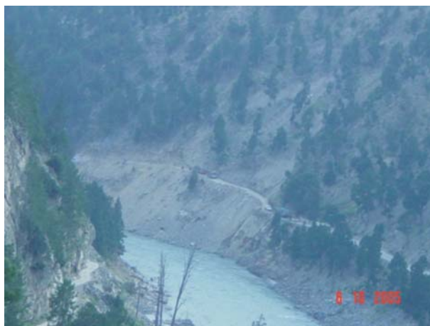
Figure 7 Shongtong landslide located about one km upstream of the Shongtong Village and affecting the NH-22.
