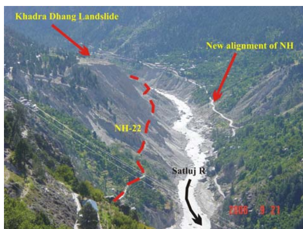
Figure 11 Khadra Dhang landslide located on the right bank of the Satluj River. The new alignment of the NH-22 on the left bank of the river, has made the entire hill slope unstable.
