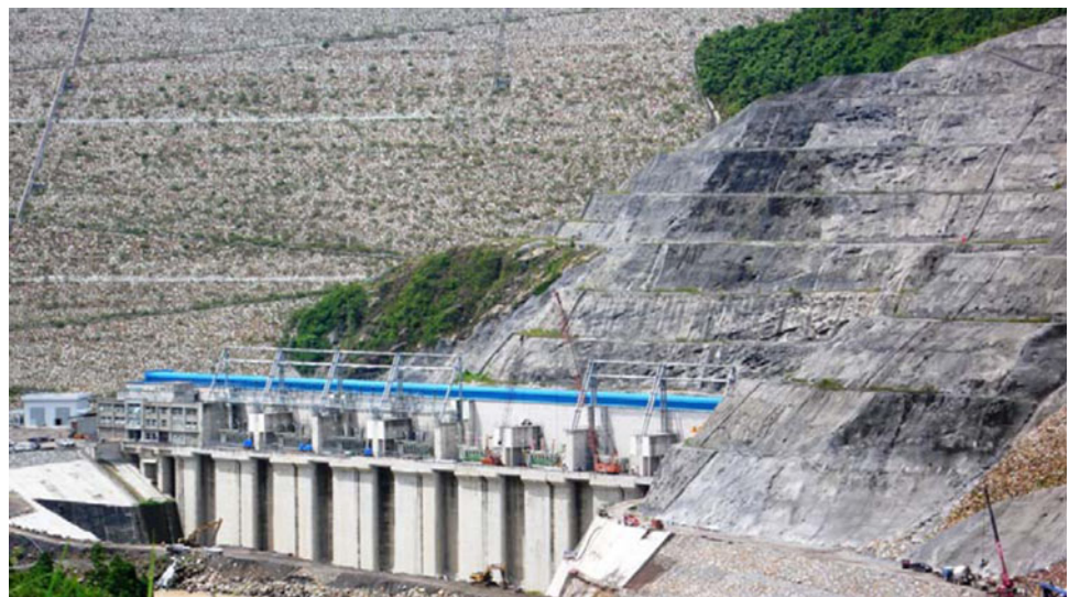
Fig. 2 The Bakun hydroelectric facility (under construction)
