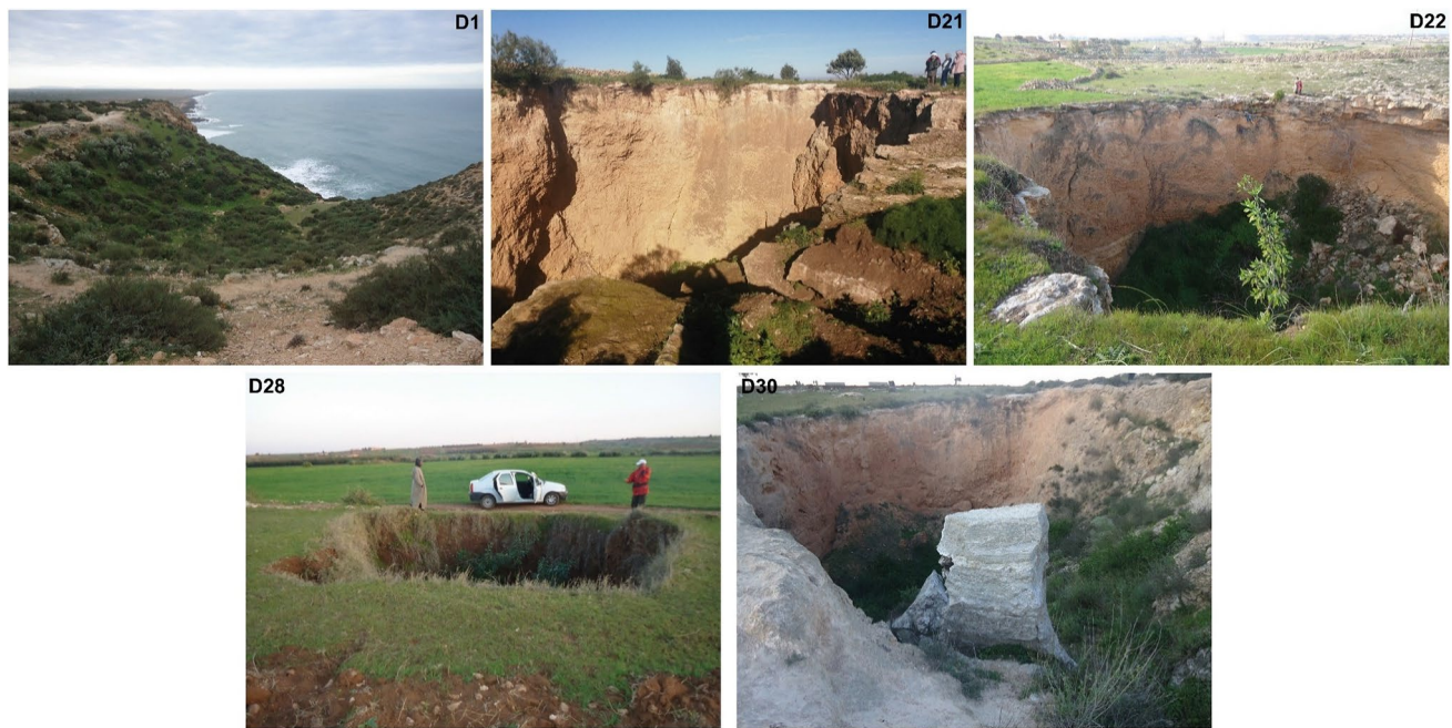
Fig. 5 Illustrative photos showing an example of collapse dolines inventoried across the study area: Dolines D1, D21, D22, D28, and D30
