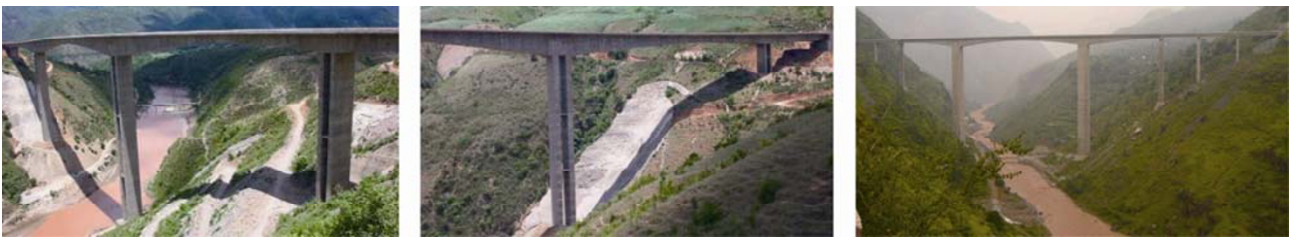
Figure 1 Typical canyon topography and rigid frame bridges.
