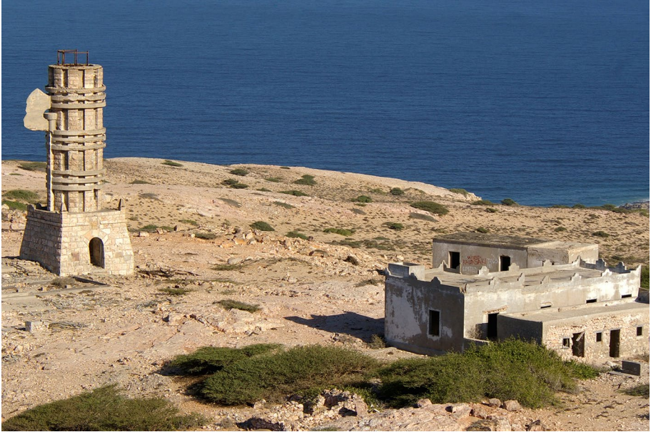
Fig. 6 Aerial view of the “Francesco Crispi” Lighthouse in 2012 (photo by A. Alpozzi)
