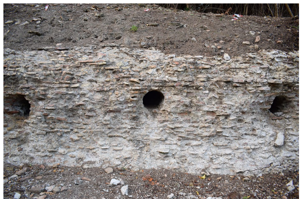
Fig. 7 Detail of the quay wall
