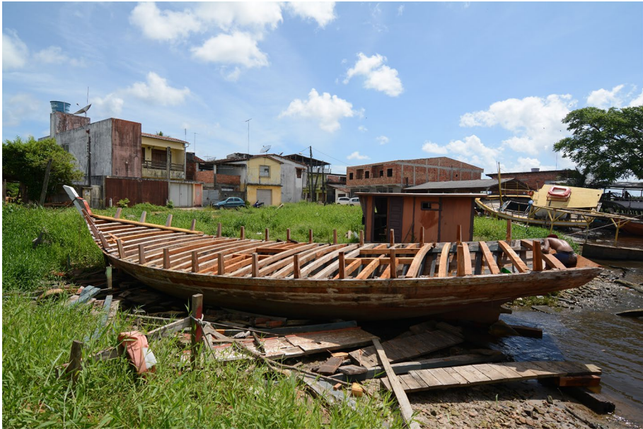
Fig. 4 Saveiro under construction in 2013 at the riverbank of Valença, Bahia, Brazil. Photograph: Rodrigo Torres
